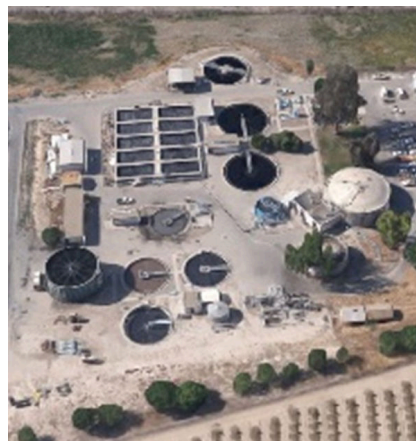
Sanger Wastewater Treatment Plant Sanger, California
