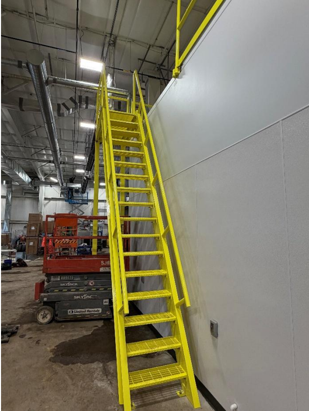
Alma Transportation Building Expansion Photos 2-6-2026
