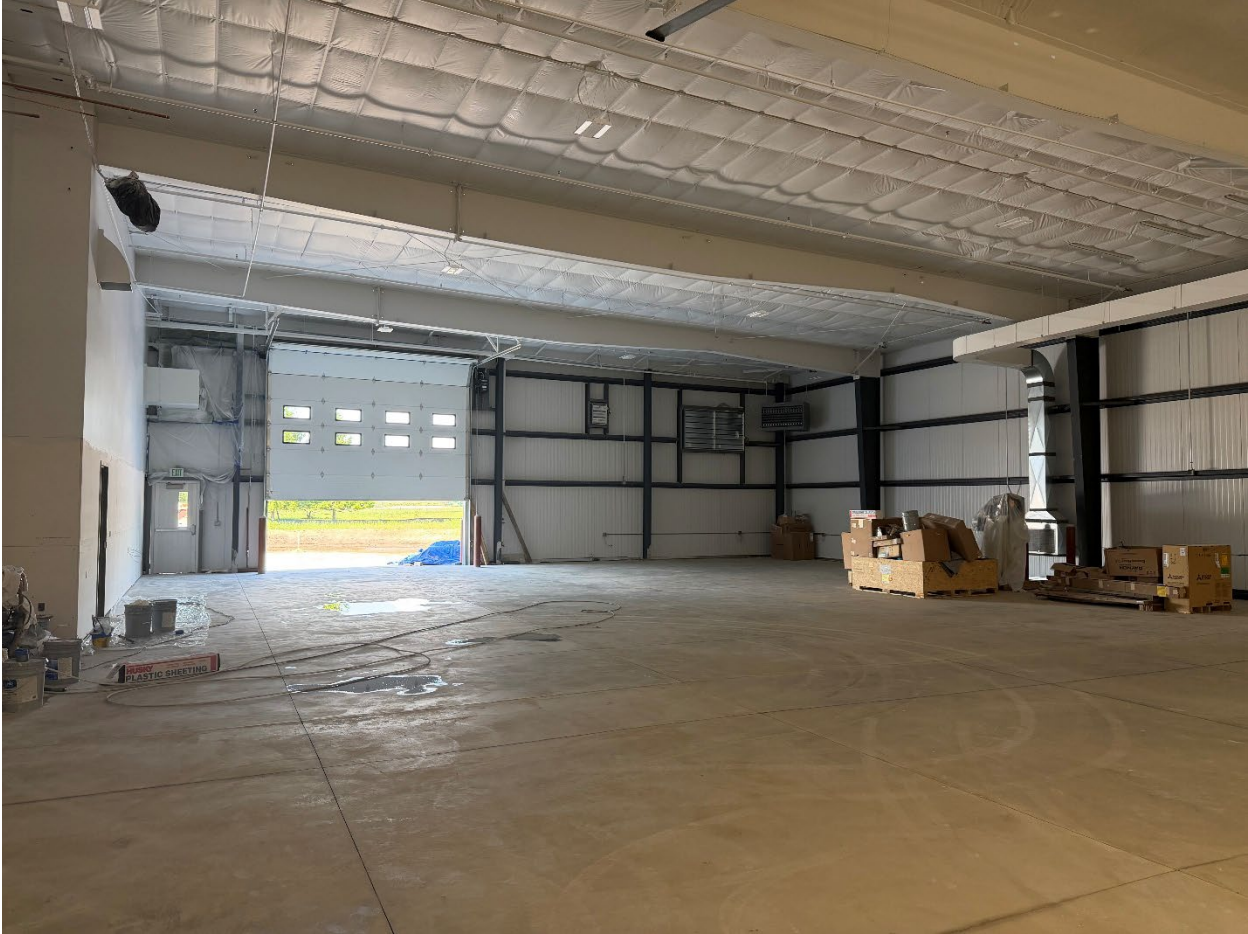
Transit Expansion Photos 5-22-2026
