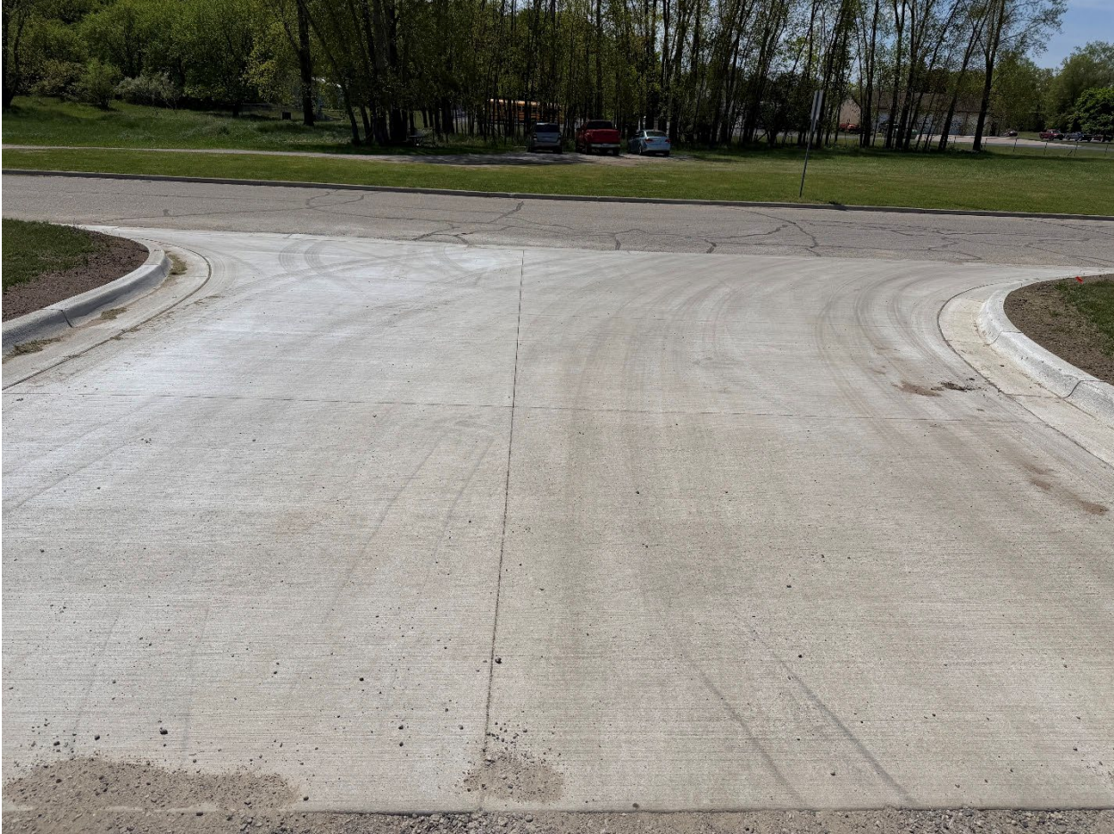
Transit Expansion Photos 5-22-2026
