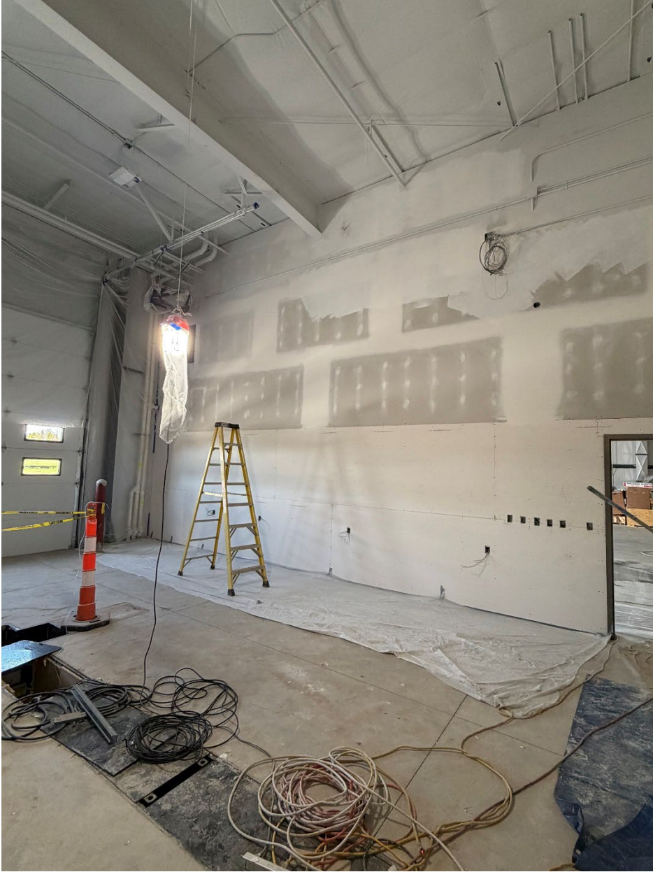
Transit Expansion Photos 5-22-2026
