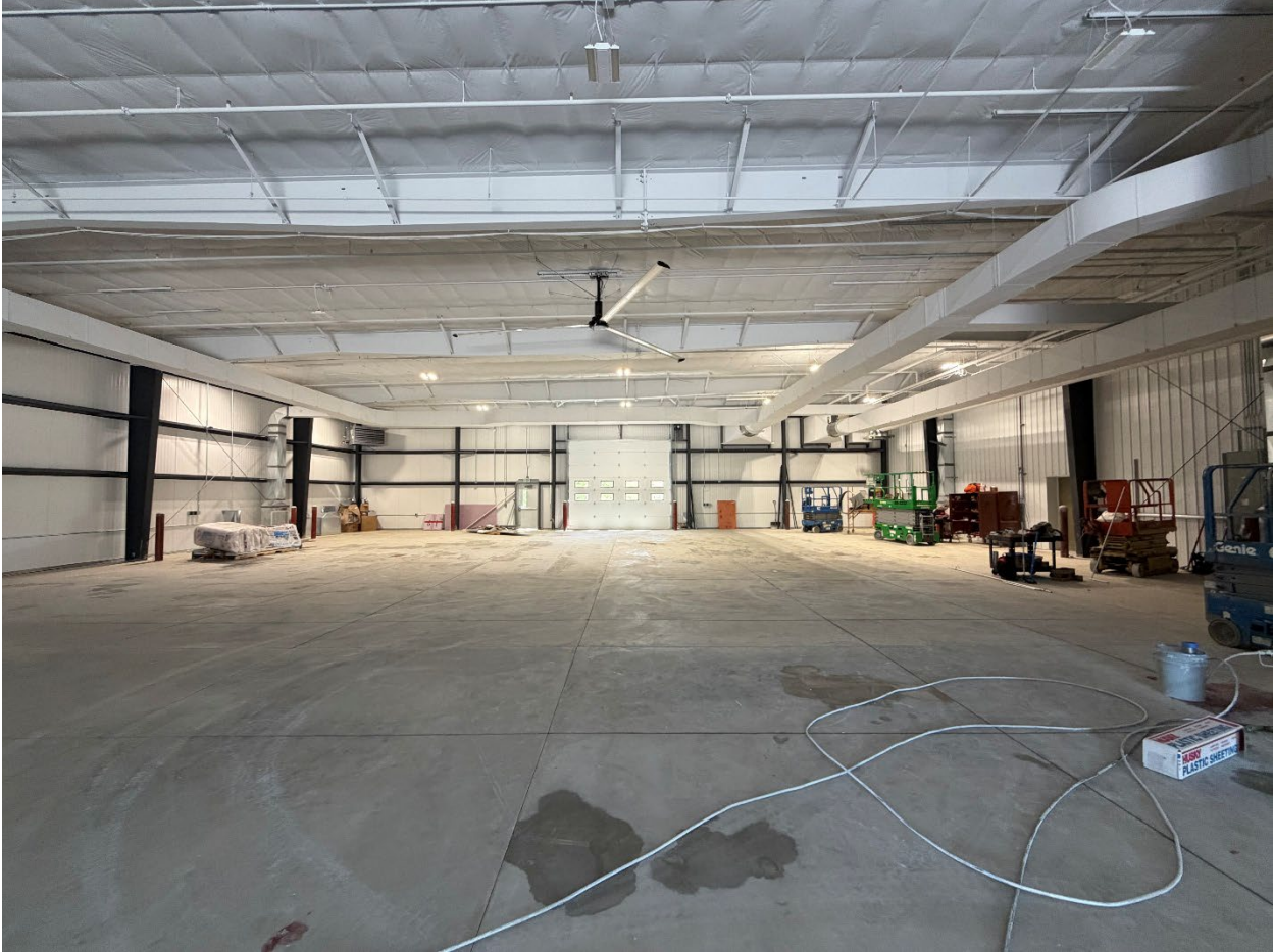
Transit Expansion Photos 5-22-2026
