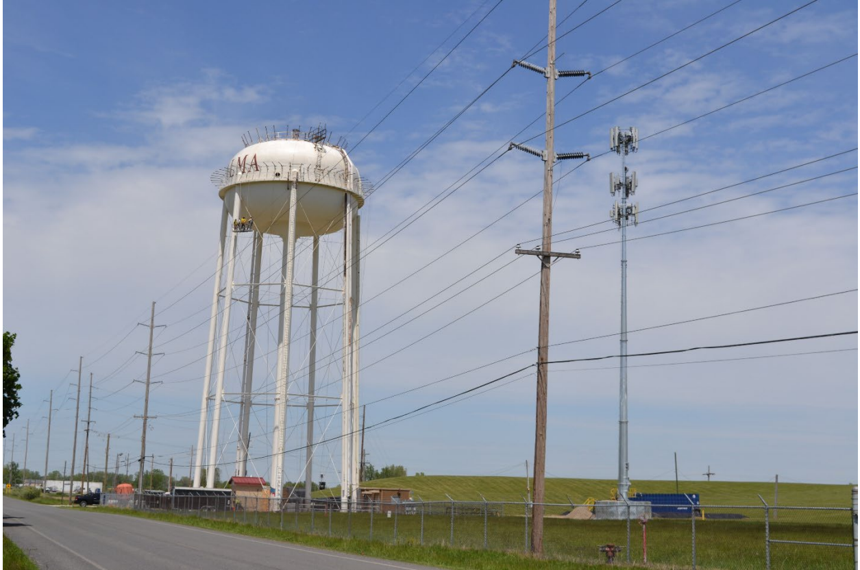
Elevated Water Storage Tank – Temporary Cell Tower
