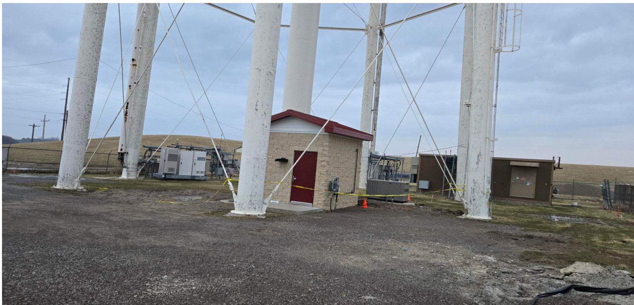
Photo #5 – Water Tower Control Building
