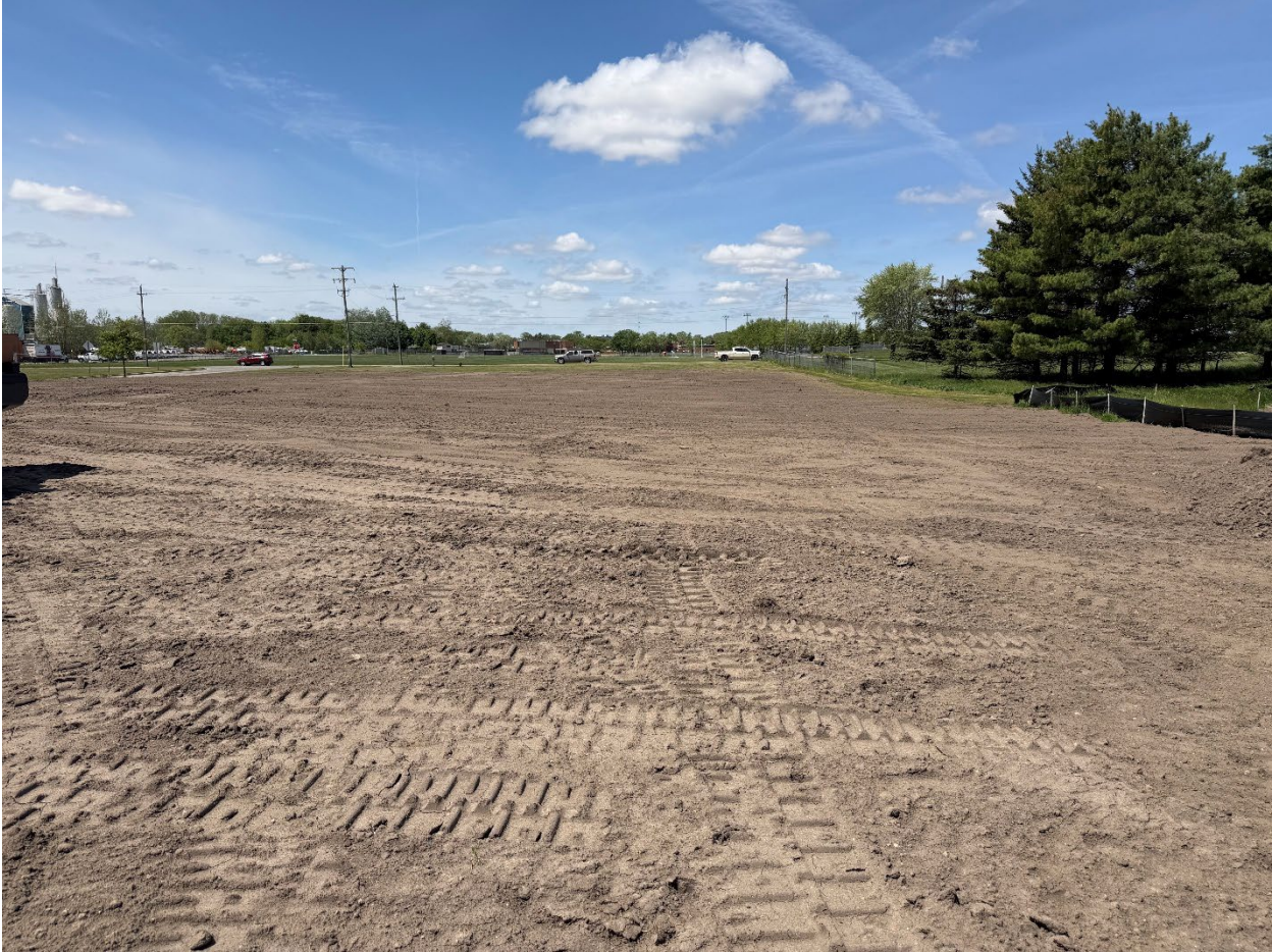
Transit Expansion Photos 5-22-2026
