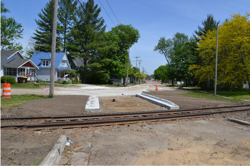
W Center Street
