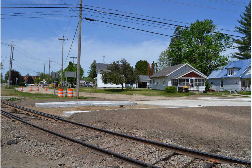
W Center Street
