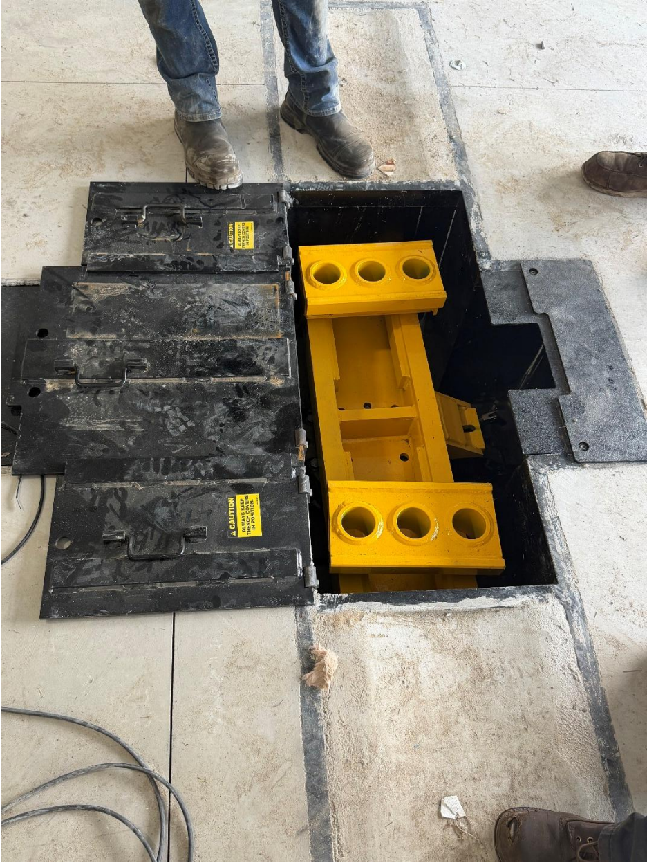
Transit Expansion Photos 6-5-2026
