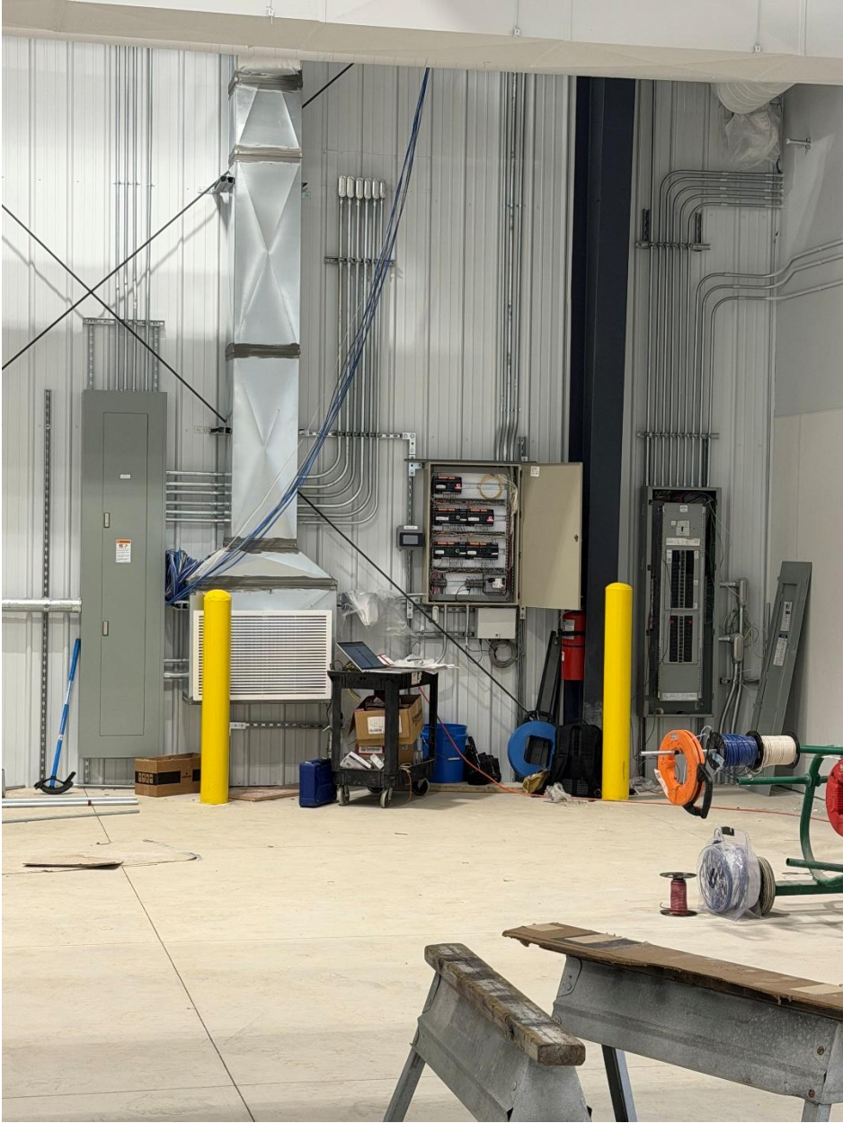
Transit Expansion Photos 6-5-2026
