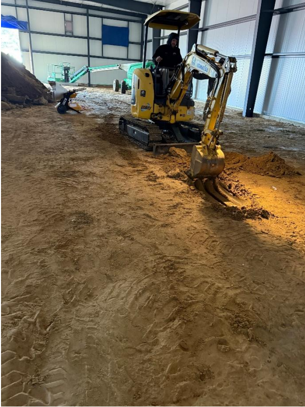
Beginning to dig the pit for the vehicle lift.
