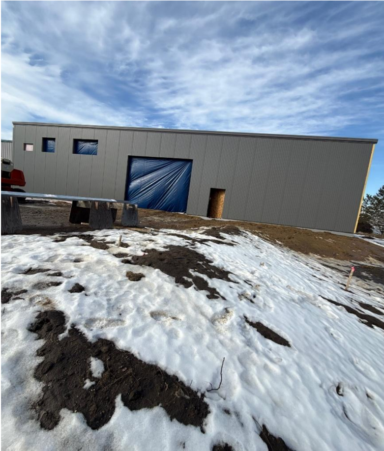
Building Addition is enclosed
