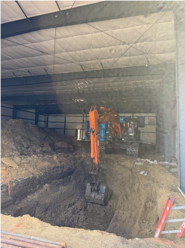
Lift Pit progress.
