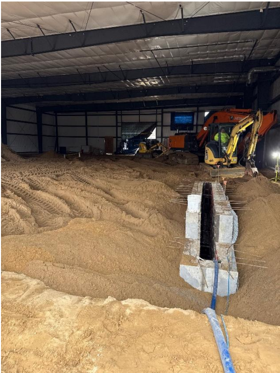
Interior of Building Addition
