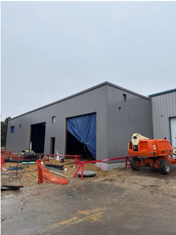
Exterior of Building Addition West Side
