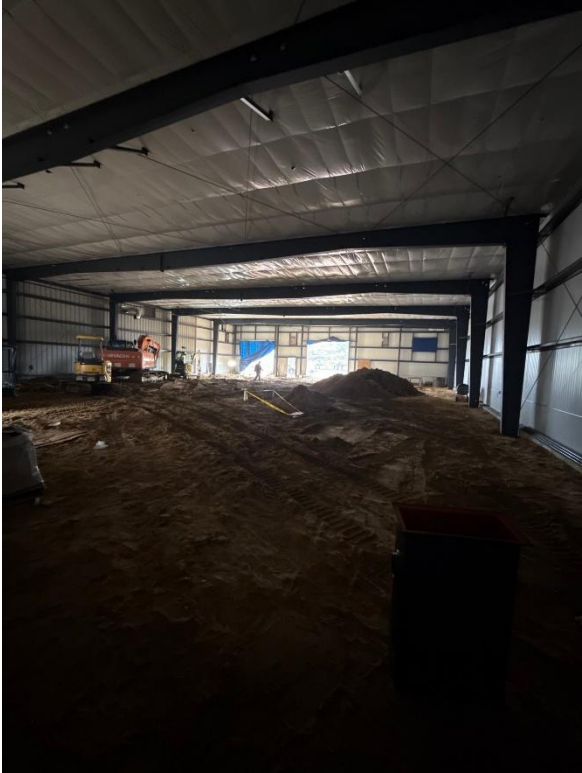
Interior of Building Addition Looking West
