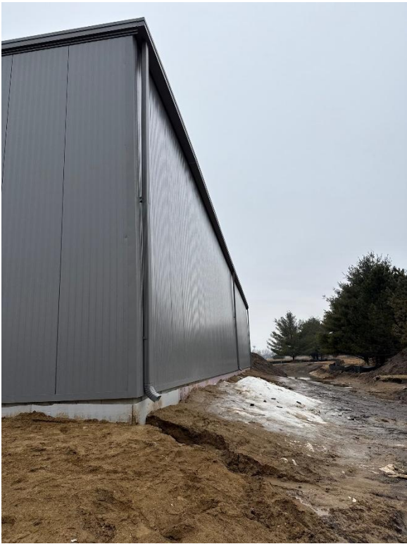
Exterior of Building Addition North Side
