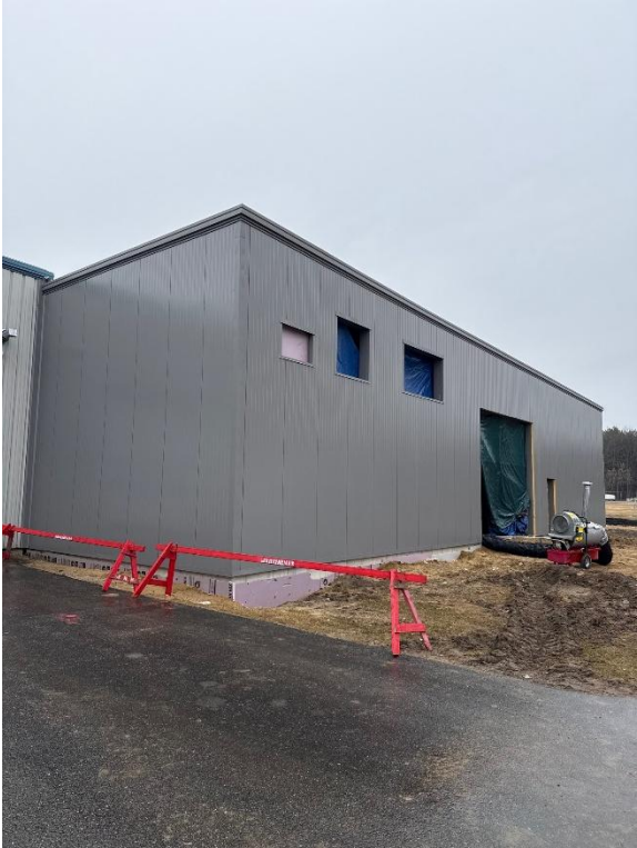
Exterior of Building Addition East Side
