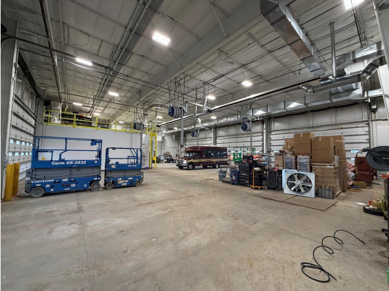
Transit Expansion Photos 3-24-2026
