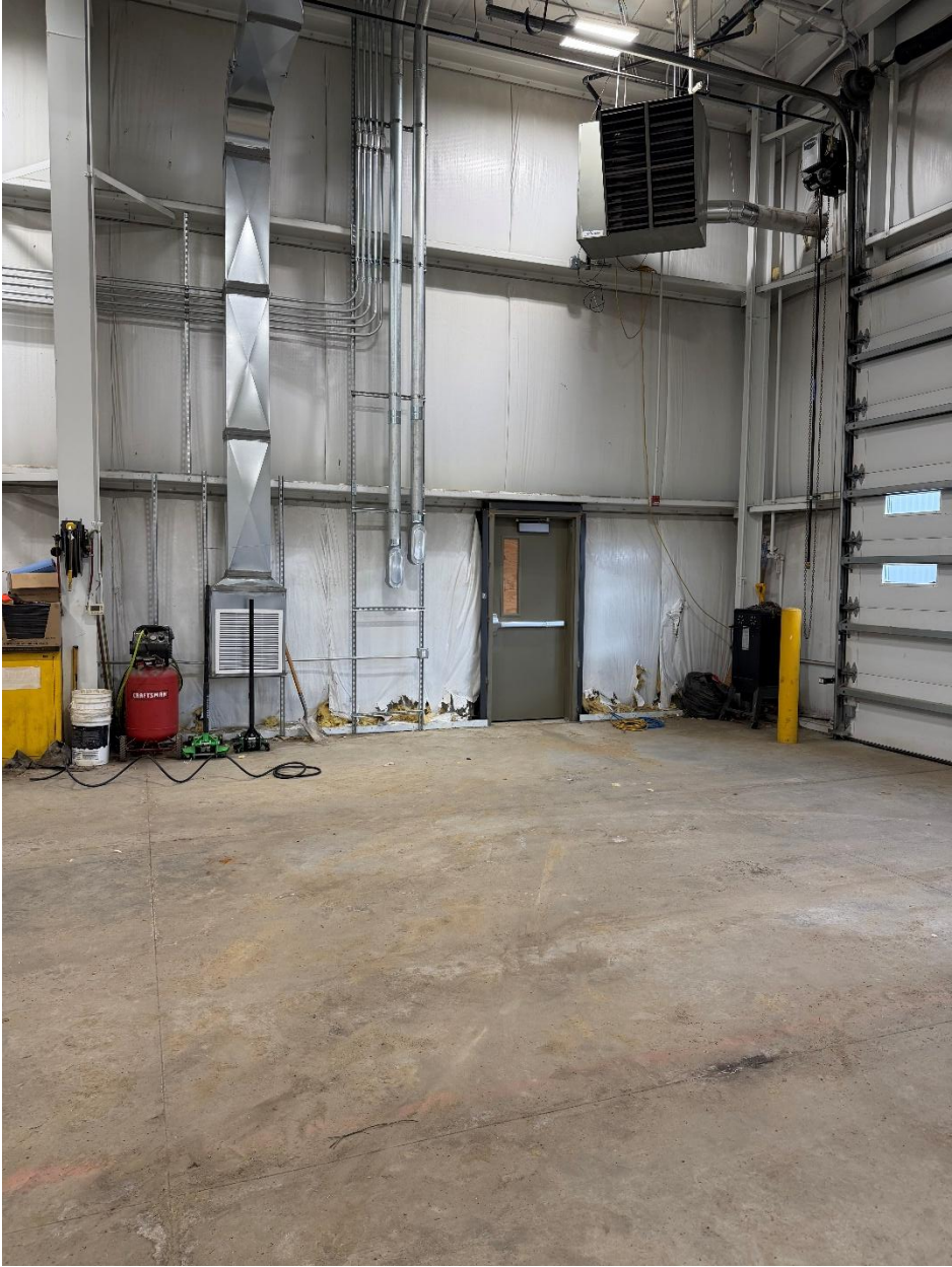
Transit Expansion Photos 3-24-2026
