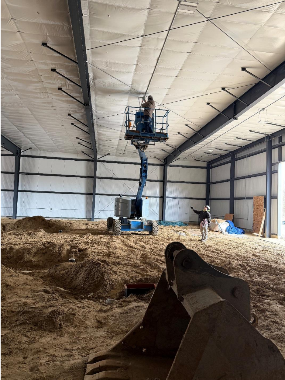
Transit Expansion Photos 3-24-2026
