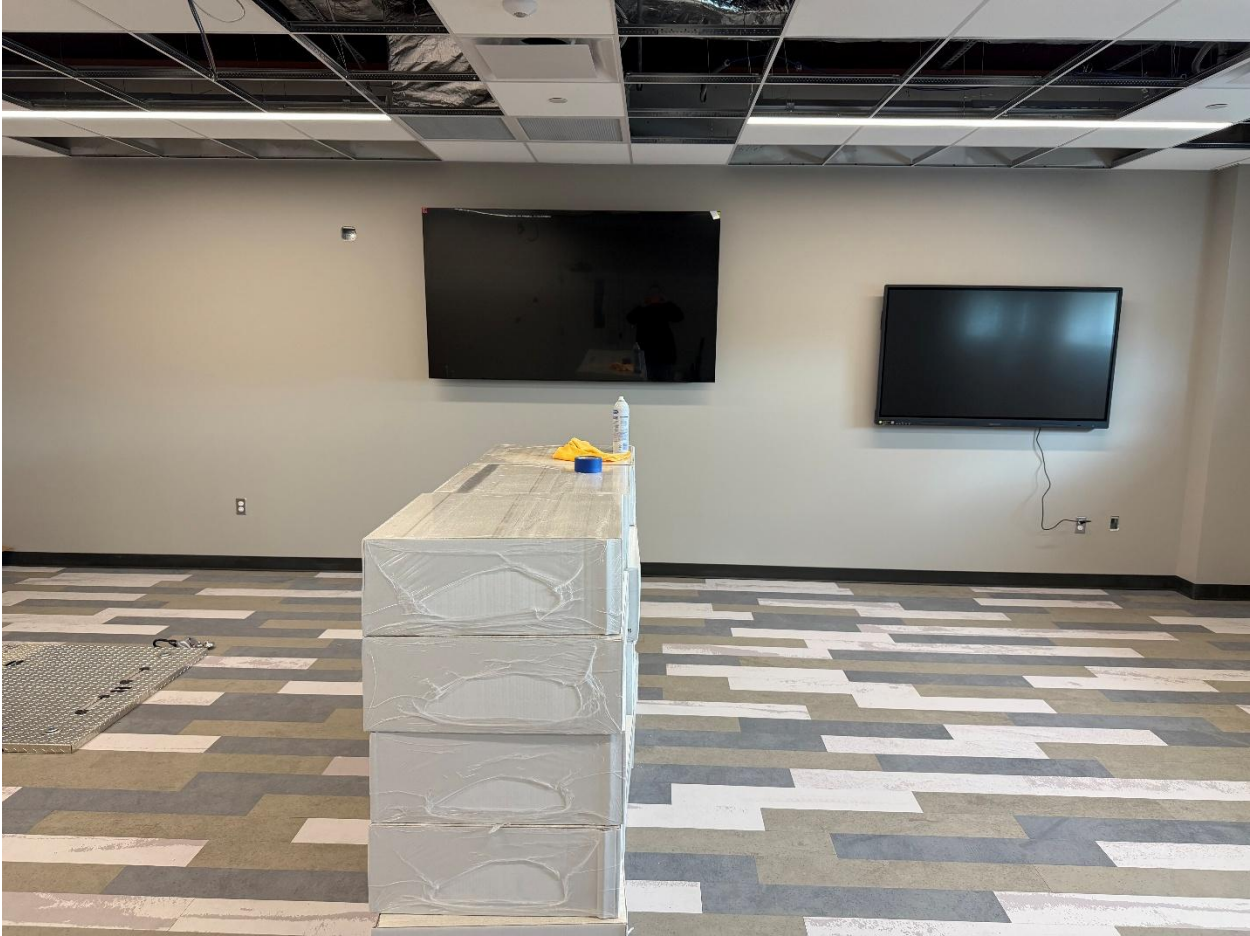
Transit Expansion Photos 3-24-2026
