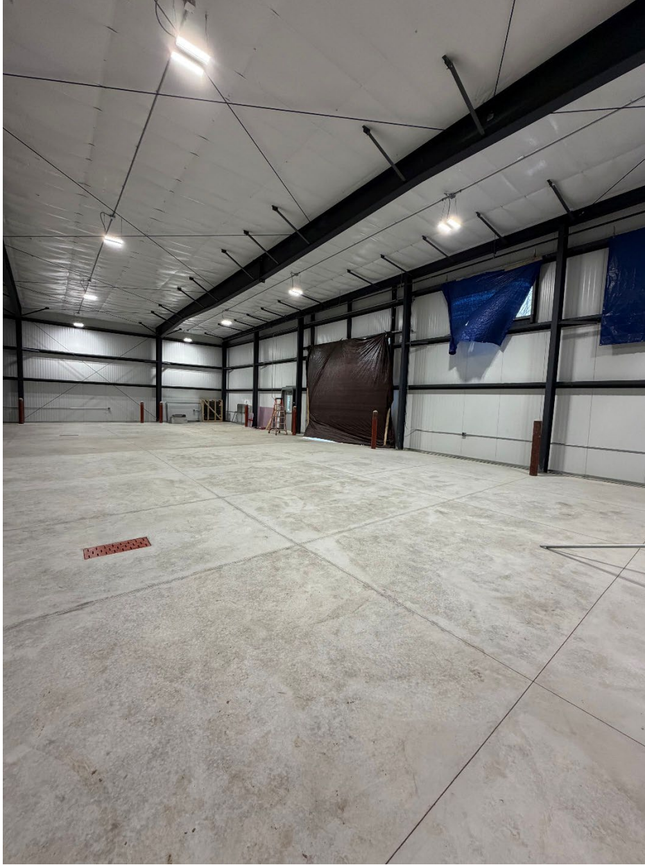
New Floor and Walls in the Building Expansion
