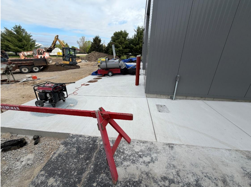
Alma Transit Building Expansion Photos 5-7-5206
