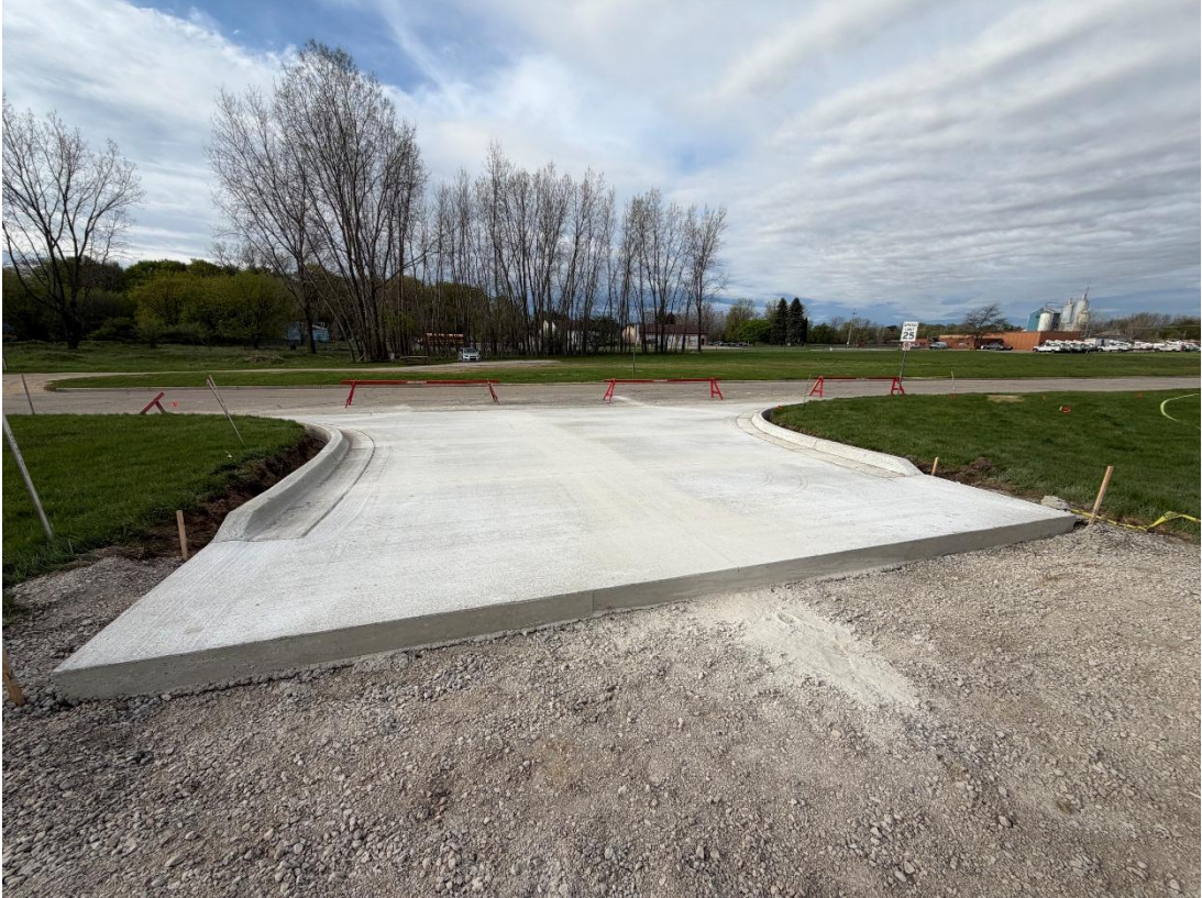
Alma Transit Building Expansion Photos 5-7-5206
