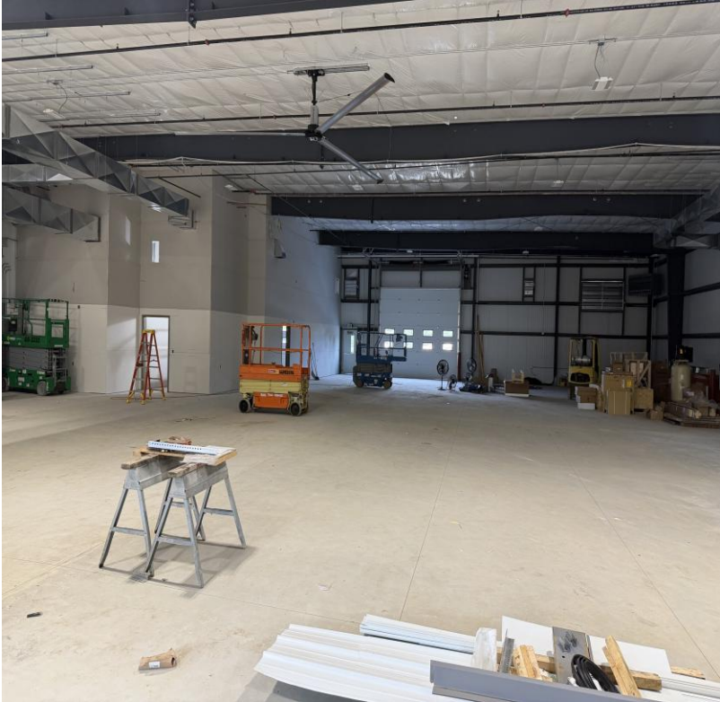
Alma Transit Building Expansion Photos 5-7-5206
